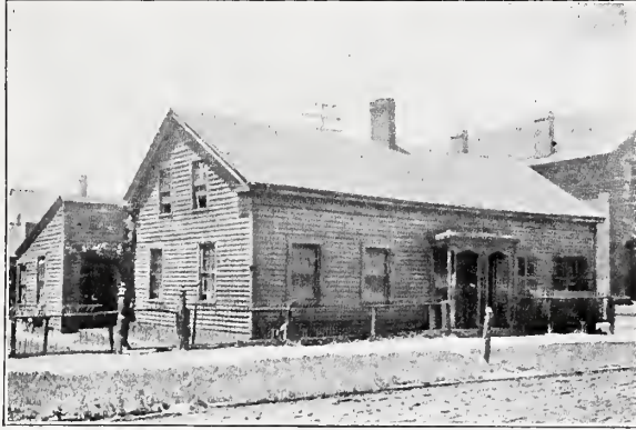
Said to be the oldest house in Cleveland, and to have been used by Astor's Fur Company before Cleveland was surveyed. There is great doubt as to this. Alfred Kelley locates a Trading House on the west side, on his map of 1814, giving date of house as 1786. This may be the house here shown. The house was built of hewn timbers, later covered with sidings. Joel Seranton owned it for a number of years and sold it to Robert Sanderson in 1844. It was moved to Frankfort street from its original location on the flats near the river. See "Annals Early Settlers' Association," No .5, p. 84.
